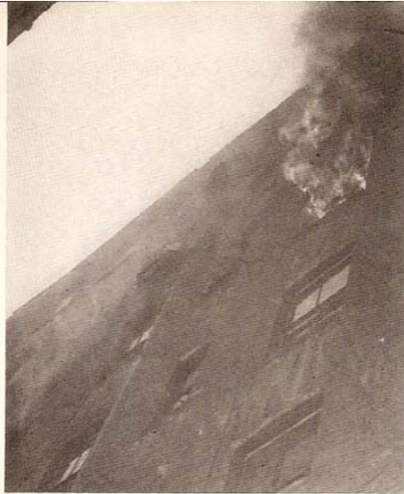
The above picture was taken a few minutes after fire broke out in Robles' apartment and while Robles was still exchanging shots with the police (right). Members of Eng. 58 and L. 26 look up at policeman on third floor reporting that fire had started. Note line ready to go.
